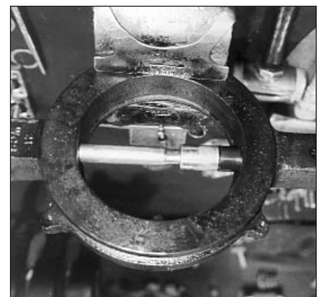
Figure 6 – Shows partial insertion of the stem bearing.
