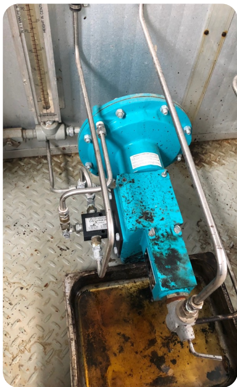
High Bleed Pneumatic Chemical Pump utilizing fuel gas as power source - methane emitting
