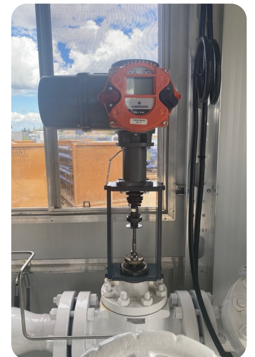
Bettis RTS Linear Fail Last Actuator on Fisher 3" HPT or Fisher ET Control Valve
