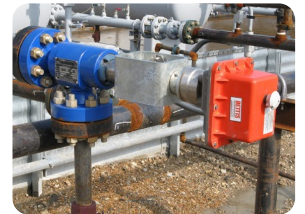
Bettis EM 500 Series Multi-Turn Electric Actuated Automated Wellhead Choke Valves
