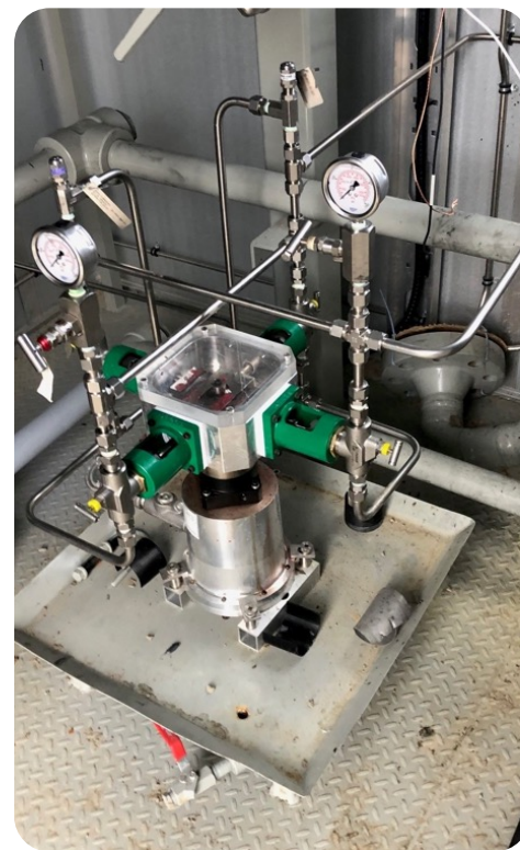
High Bleed Pneumatic Chemical Pump utilizing fuel gas as power source - methane emitting
