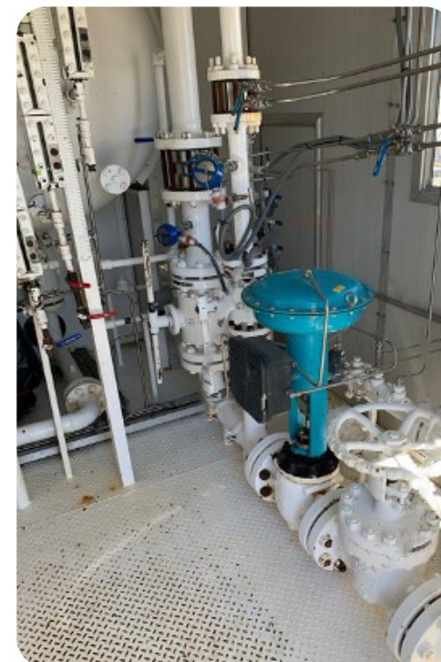
Bettis RTS Linear Fail Last Actuator on Fisher 3" HPT or Fisher ET Control Valve
