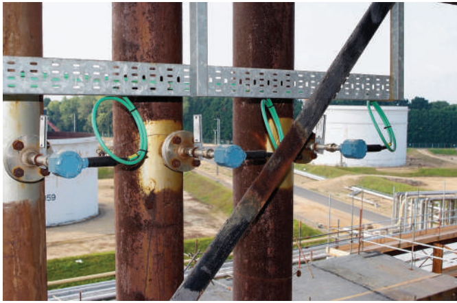
Figure 3-81: Thermowell Installation Examples
