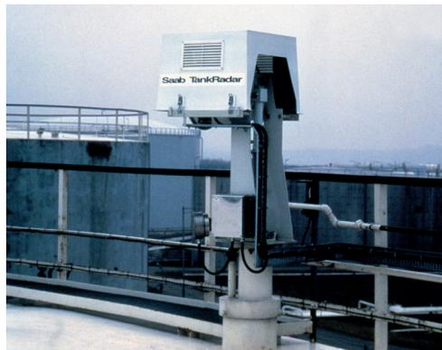
Figure 2.9: First high precision radar gauge installed in 1985 on a refinery tank.
