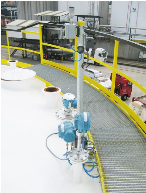
Figure 9.8: Antenna connected to tank devices.
