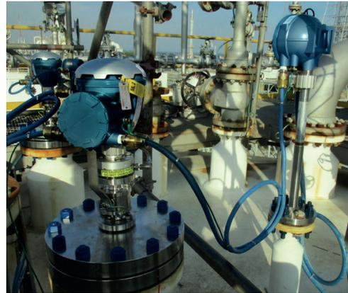
Figure 9.3: Tank redundancy is accomplished with dual tank gauges and separated communication layers - wired and wireless.
