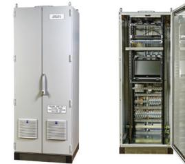
Figure 9.5: A tank gauging system cabinet.
