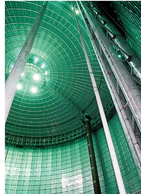
Picture 7.4: Full containment tank used for storing refrigerated liquefied gas.
