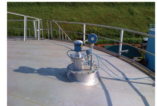
Figure 3.4: Manways are normally located near the tank wall which provides mechanical stability.
