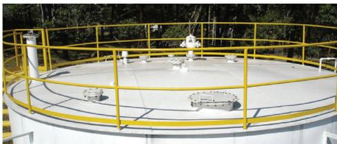
Figure 2.14: Fixed roof tank openings.
