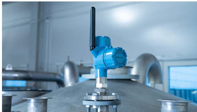
Rosemount 3408 Wireless Non-Contacting Radar Level Transmitter
