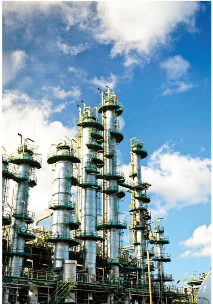
Figure 1. Distillation columns
