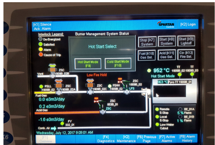
Standard HMI local control
