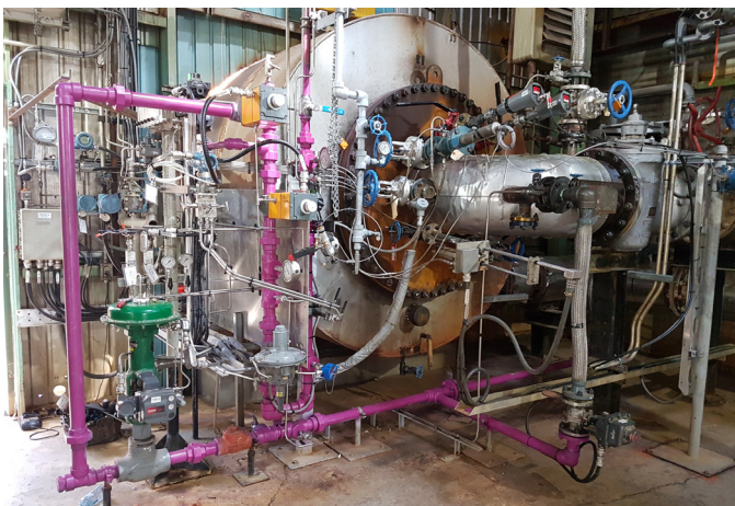
Reaction furnace (acid gas)
