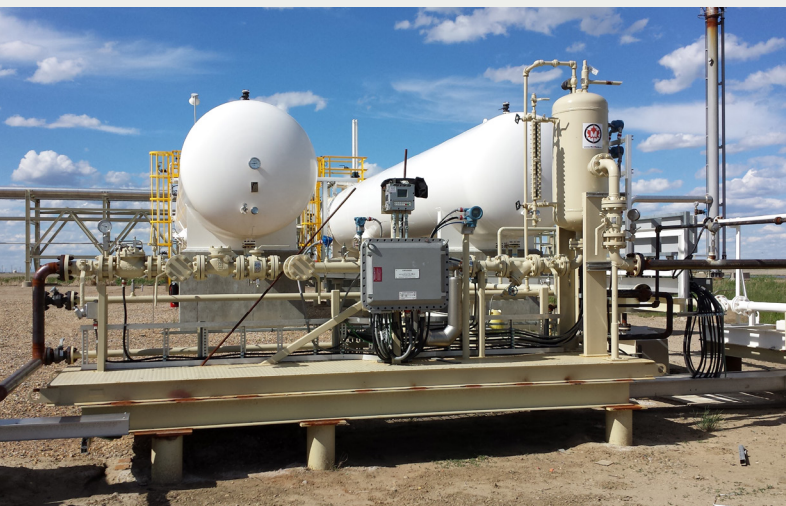
TruckVue™ NGL Transfer Point
