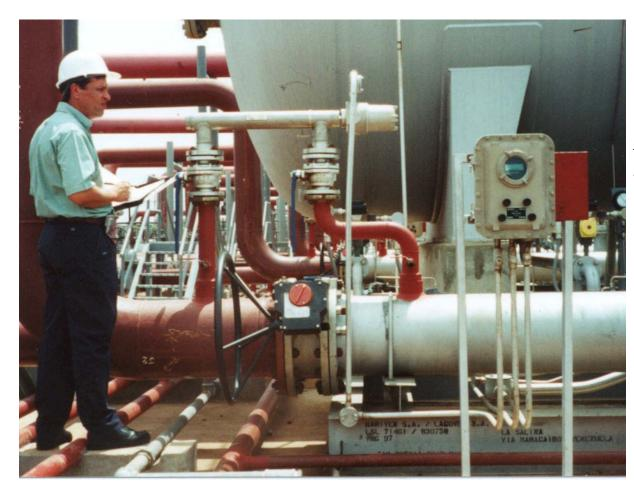
This Mounting Allows Gas or Oil to Build up In the Analyzer Unless The Flow Rate is High Enough to Flush it Through
