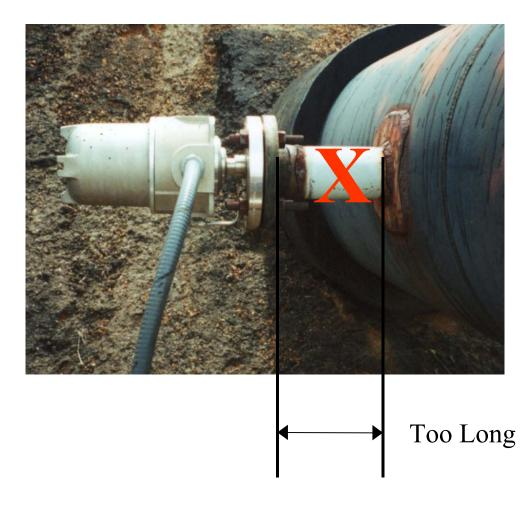
This Mounting Has Too Long of A Distance Between Pipeline and Flange - Insertion Analyzer Does Not See Main Flow
