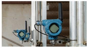
• The AMS 9420 delivers critical vibration information directly to the control room to help operators identify potential production risks.
