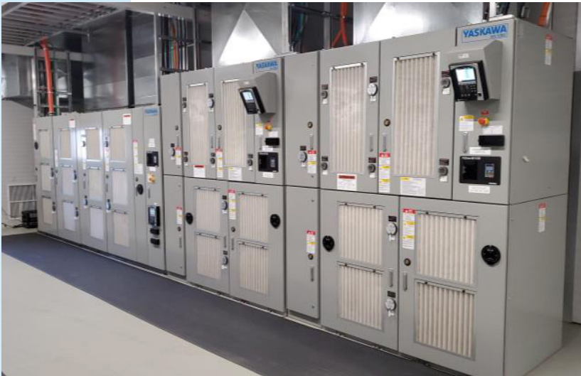
Spartan Controls Yaskawa MV1000 VFD
