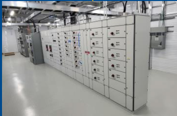
PowerVue™ Motor Control Centers
