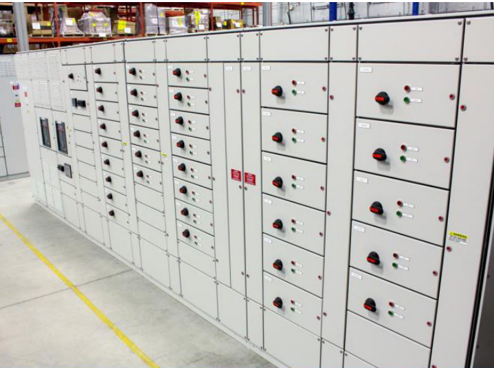
Spartan Controls PowerVue™ MCC with ATS and DeltaV™
