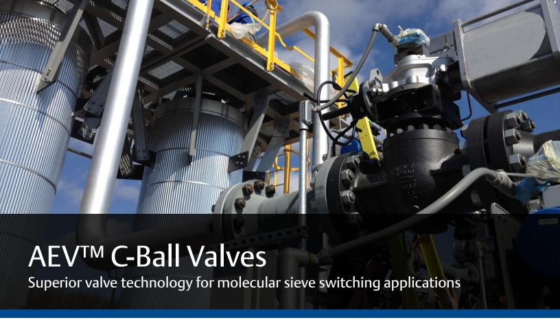
Using rising stem designed valves for switching on molecular sieves presents a real challenge with seat wear and leakage coupled with the ongoing maintenance required to meet stringent regulatory emission requirements. There must be a better solution.
