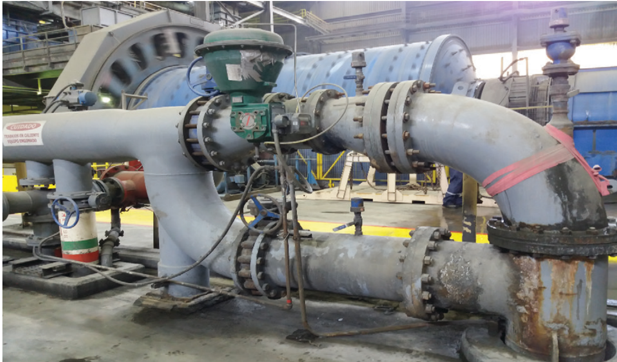
Figure 3: Recycled water feeds to the mills and screens usually require large port valves, like this Fisher V300 with stainless bodies and hardened trim, to handle the entrained particles.
