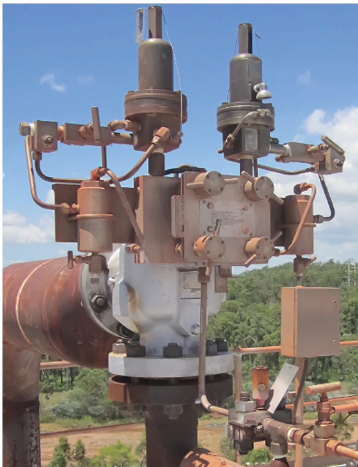
Figure 5: This redundant pilot Anderson Greenwood 500 series relief valve is installed on an alumina digester. The steam purged installation reduced downtime and saved significant costs over the previous rupture disk arrangement.
