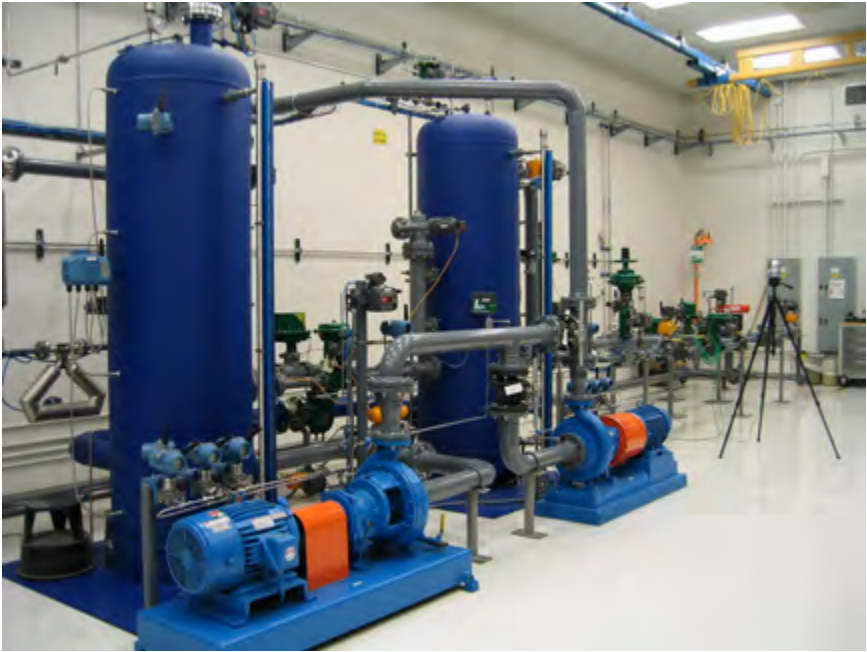
Figure 2.2 Performance Test Loop
