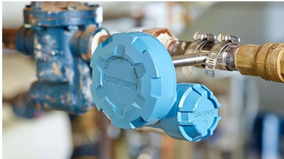
*Figure 3.3: Emerson's Rosemount 708 Wireless Acoustic Transmitter gathers data on steam trap operation and sends it to a data analytics application to determine proper functionality.*
